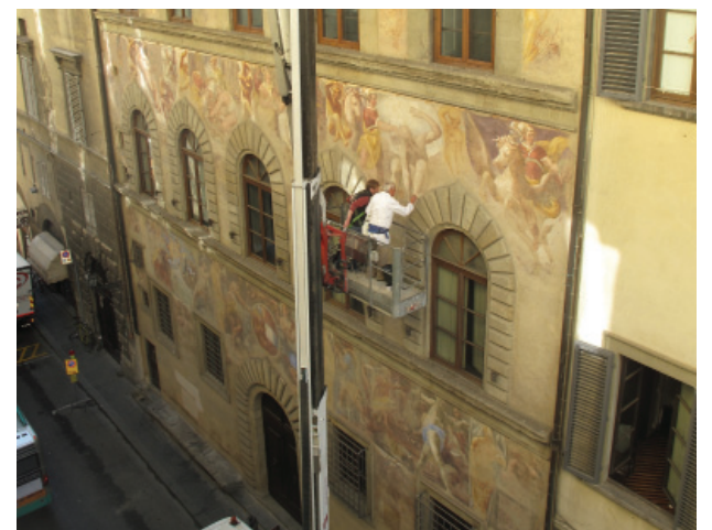
Fig. 3: Palazzo Mellini-Fossi (Florence, Italy): Examining readhered paint-layer flakes with Sabino Giovannoni who realized this ethyl(poly)silicate-based readhesion intervention on the façade in 1994 (Photo: Francesca Piqué).
