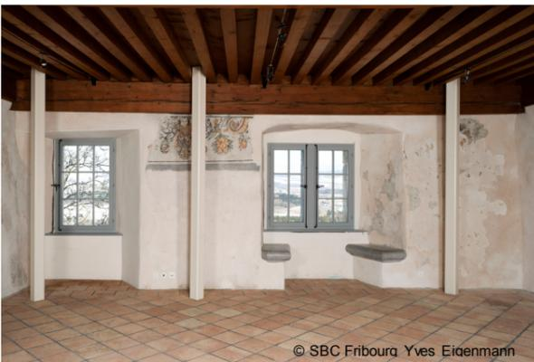
Fig. 1: North west wall of the "Salle de la Bourgeoisie" of Foyer St Germain in Gruyères. The North corner (on the far right) shows severe plaster detachment following water infiltration.
