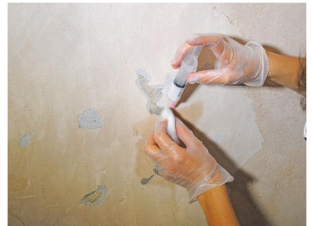
Fig. 3: Treatment trials using *CaLoXiL* injection-grout to re-adhere the detached gypsum finishing plaster.
